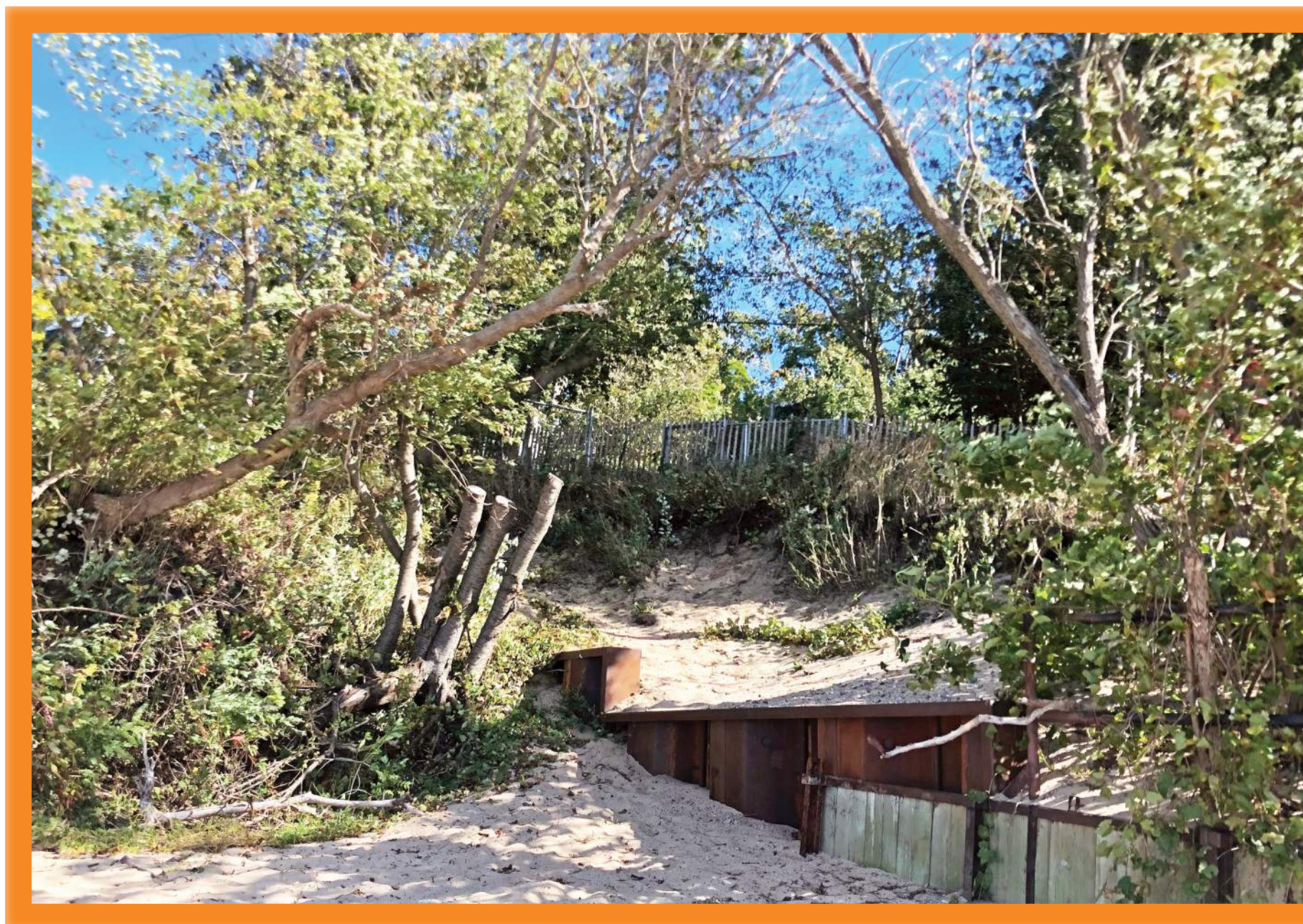
F. Slope erosion is apparent along north original park property line.
