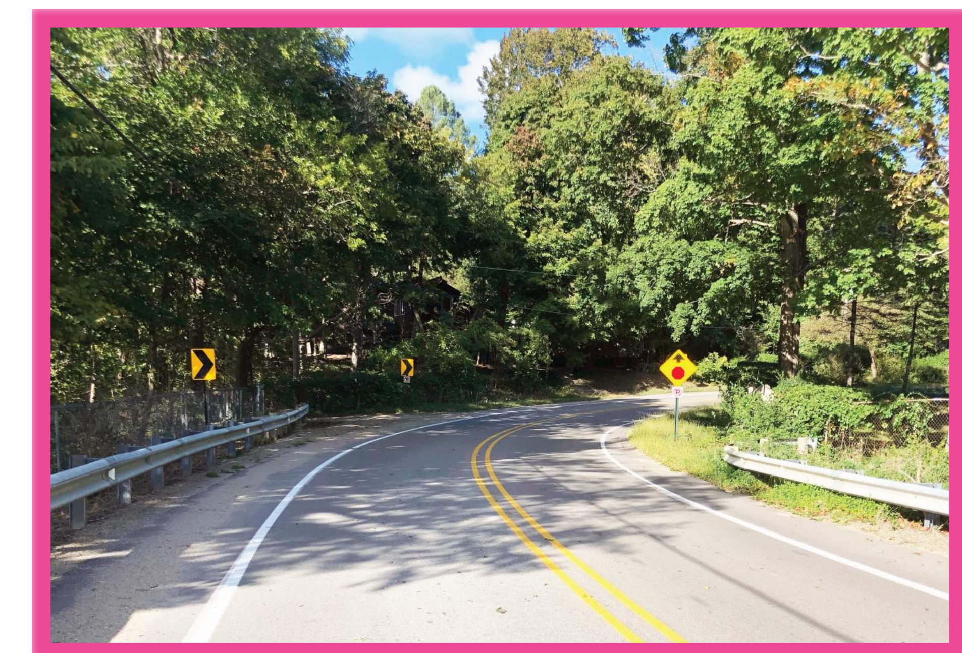
L. Pedestrian travel along east roadway shoulder is less safe due to limited sight distances. Road shoulder may be modified to accommodate pedestrian use. Metal guardrail may be replaced with more aesthetically appropriate guardrail.
