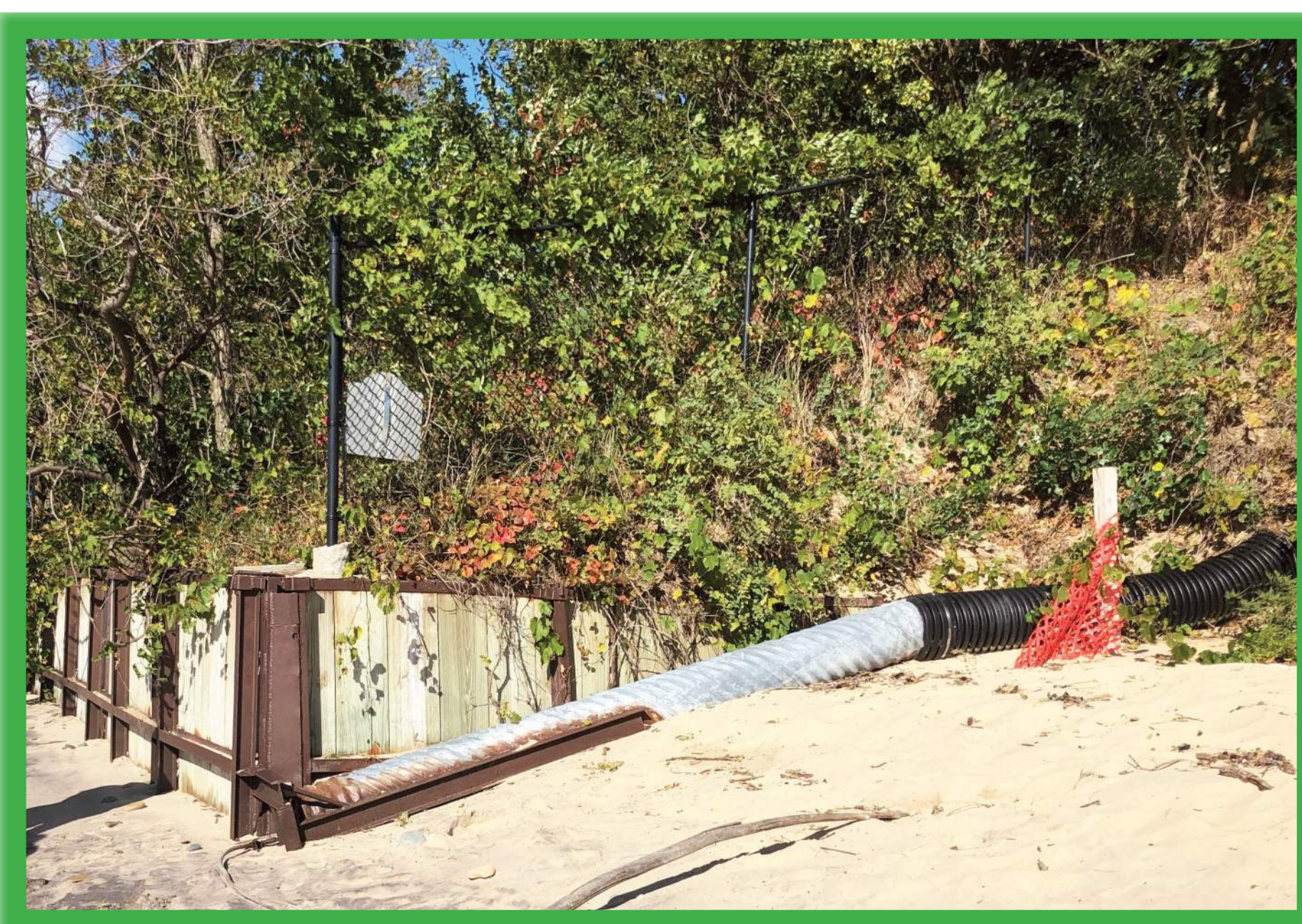
I. Steel and wood seawall should be monitored to address maintenance needs. Potential to improve aesthetics by addressing stormwater outlet.
