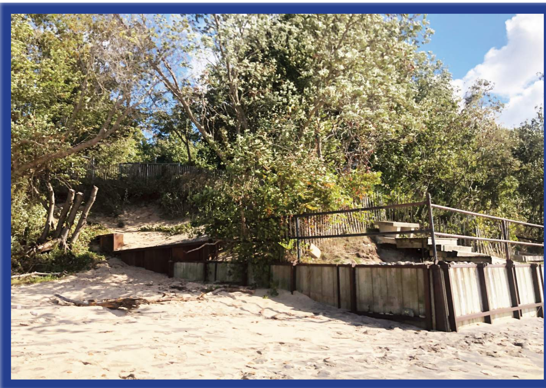
E. Grade is retained by a combination of shoreline retaining walls, and existing vegetation. Terracing provides overlook space.
